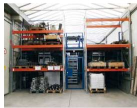
META QUICK<sup>®</sup> shelving system optimally integrated with the room, with prefitted META MULTIPAL<sup>®</sup> pallet racking system and loading station
